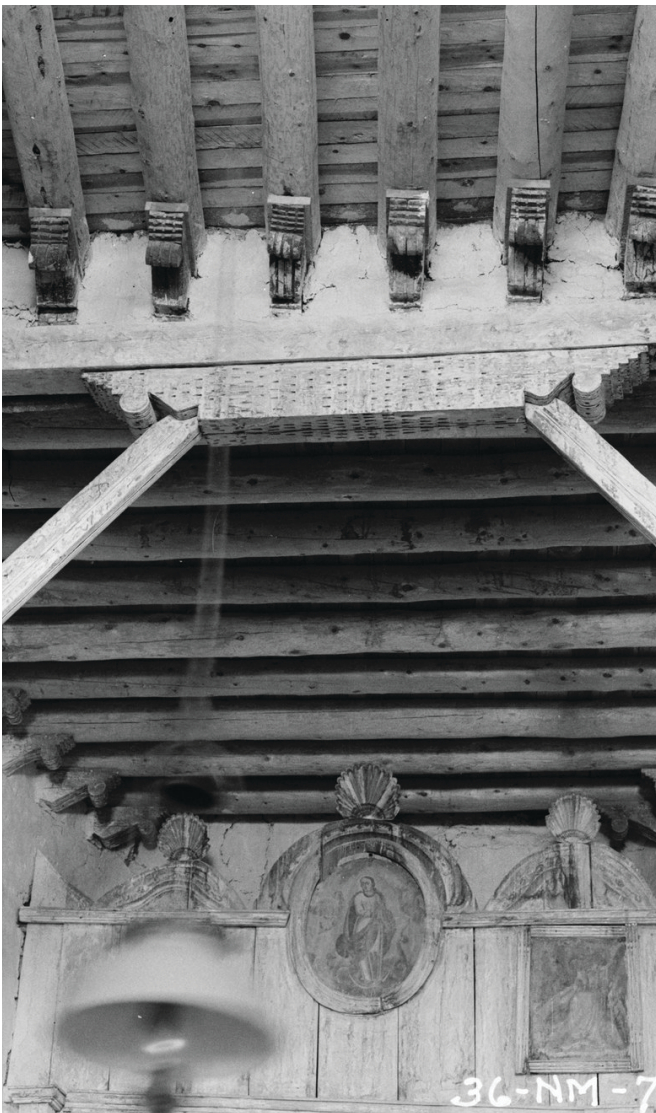
Vigas and latillas in the ceiling of San Francisco de Asis Mission Church, Ranchos de Taos, New Mexico
